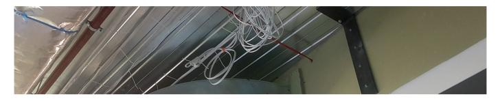
The StrongArm bracket was the perfect solution for this type of installation. StrongArm was fixed directly to the concrete structure and the hung wall, securing the installation whilst the lower wall was installed. Upon the completion of the entire wall, these brackets remained installed without the screws used for fixing to the hung wall. This process meant that the entirety of the hung wall remained supported, and the acoustic properties of the wall restored.
