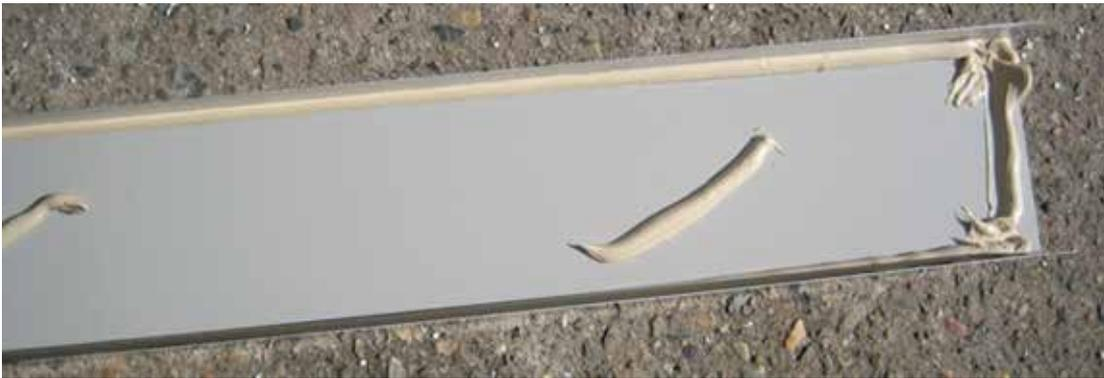
Note that the capping channel will be slightly shorter than the panel. Start at one end of the panel, approx 5mm in and carefully ease the capping channel over the panel. Once fitted, tap the capping channel to make sure it is seated correctly.
