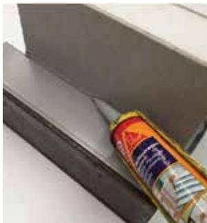
4. Apply bead of Sika between the edge of the UB flange and the UB infill.
