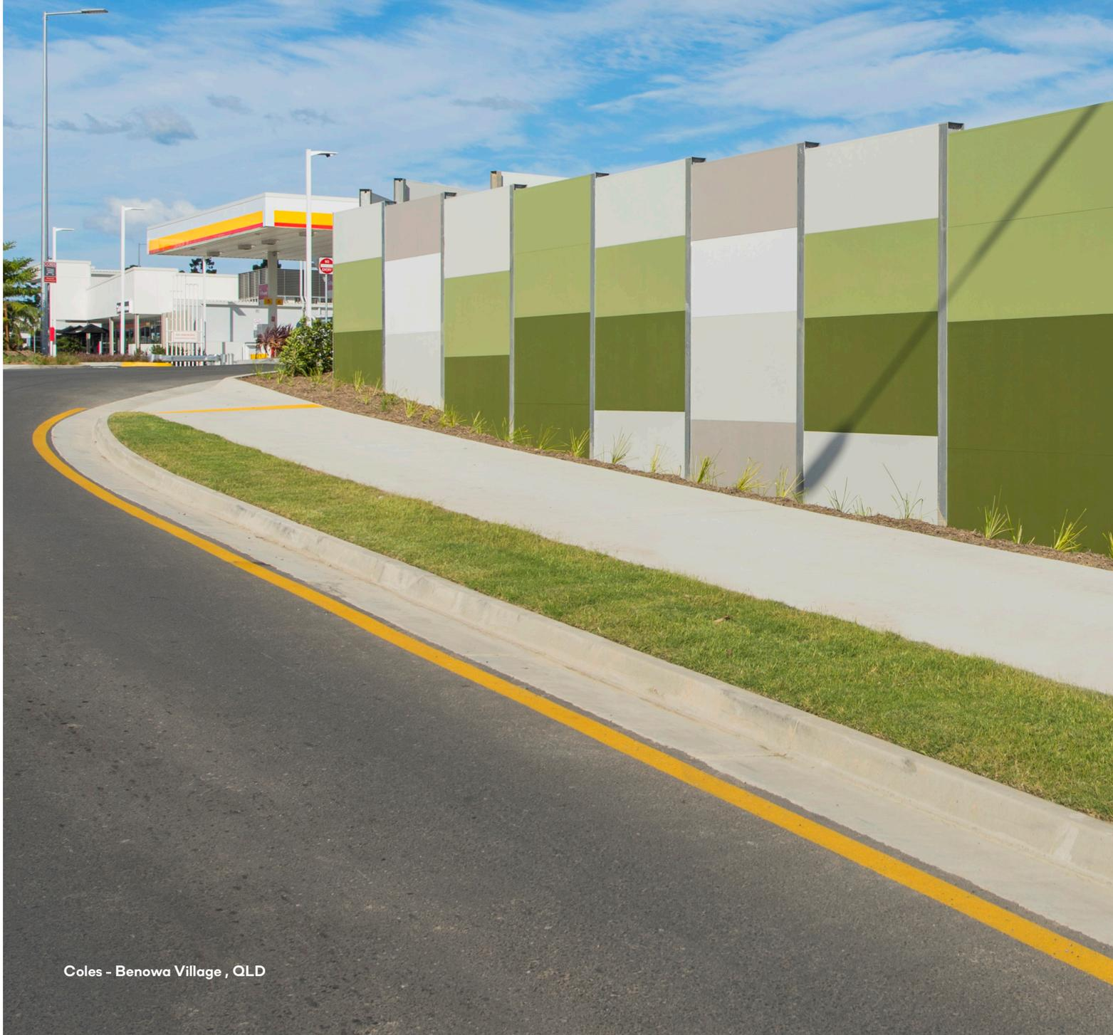
GuardianWall is designed to be a very aesthetically pleasing modular noise wall, offering privacy, security, noise abatement and rapid construction times compared to other industry noise wall alternatives. GuardianWall's most common application is as a noise attenuation wall, acoustic wall or fence, estate boundary or security wall.
