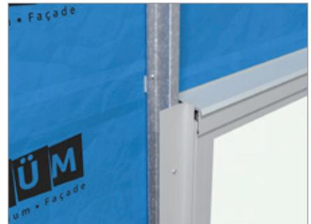
Install the vertical trims for the cladding, at the left and right of the cladding section, at either side of any wall penetrations, and at any corners. When installing down to an adjacent flat surface such as a garden bed or pathway, a minimum of 150mm from the ground is recommended to prevent rain splash back dirtying the façade.
