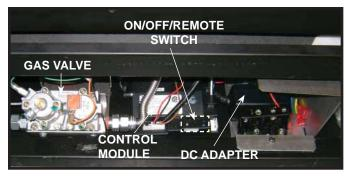
Figure 11.1. Valve Components
