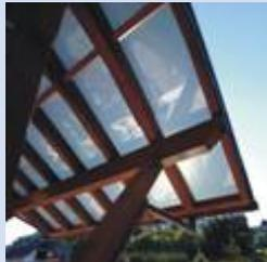
For carports or train stations, glazed roofs without a thermal insulation function are typical applications for semi-transparent laminates. It is possible to combine non-transparent ASI® OPAK areas with semi-transparent ASI® THRU areas.
