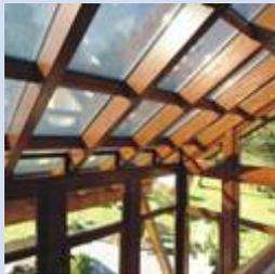
SCHOTT ASI® Glass – double glazing used in overhead application
