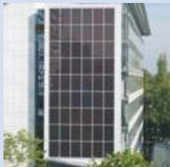
The non-transparent (ASI® OPAK) laminates can be used for rain screen cladding as well as for facades using transom and mullion systems.
