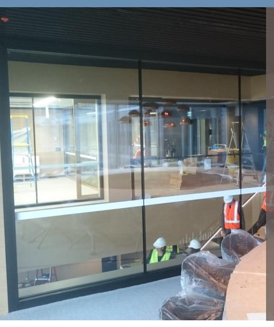
Visioneering<sup>™</sup> EI60 frameless glazed partitions is for flush-glazed interiors allowing it to blend into the surrounding architecture. Visioneering<sup>™</sup> offers the most advanced safety glass features together with a high degree of design flexibility.
