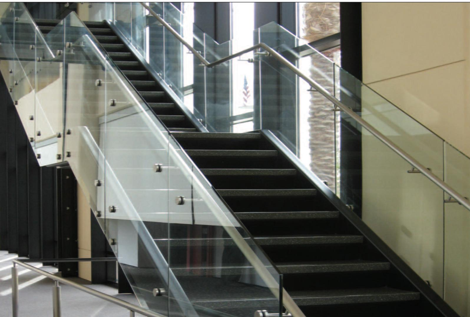
CRL is now manufacturing Standoff Railing Systems. By specialising in the design and manufacturing of this innovative system, we offer you the ability to create custom railings that will address project-specific criteria. Rest assured that the products we offer will represent the current evolution of the railing industry because product development is an ongoing process at CRL.
