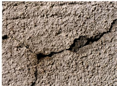
Weathered and deteriorated masonry structures have long represented one of the most difficult maintenance challenges for the contractor. In the past five years, recoating with an elastomeric wall coating has become one method for repairing these surfaces.
