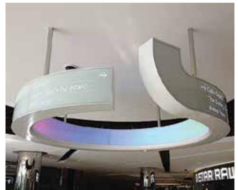
6mm Amiran low iron anti-reflective double coated toughened curved glass
