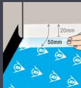
Ensure that the perimeter of the installation is sealed with waterproof tape, running the tape at least 20mm up the walls.
