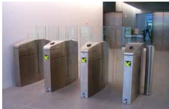
MPH - Retractable Barrier in a company foyer
