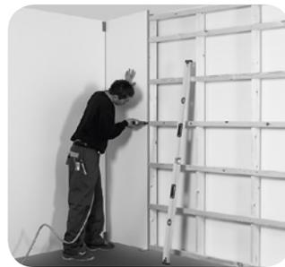
3. Fit the notches of the Clip profile (every 400mm).
