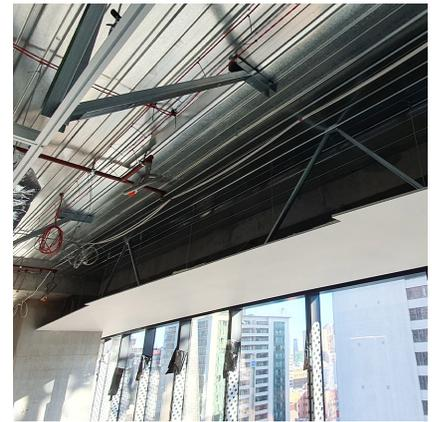
Engineering challenges also provided opportunities for collaboration. Working closely with Kusch consulting engineers, intricate ceiling designs could incorporate a seismic design without compromising on necessary utilities running throughout the ceiling. This collaboration could then be applicable throughout multiple areas of the project.
